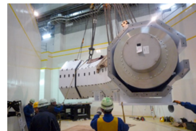
curved solenoid installation
